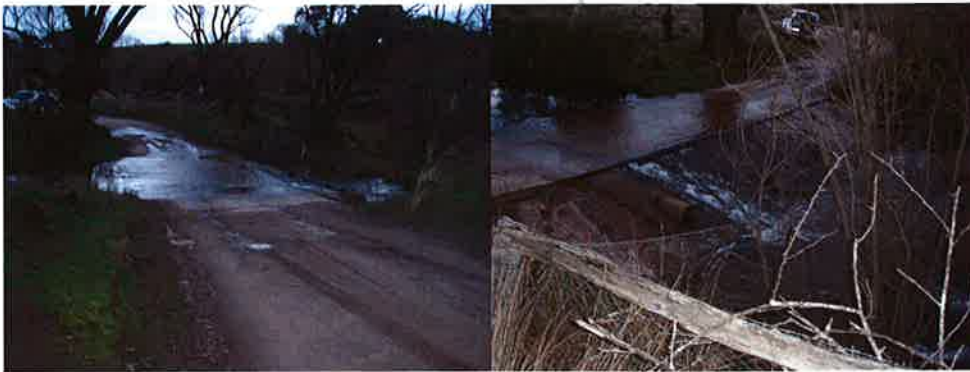
Figure 10: Views of the road crossing on Wiaborough Creek
